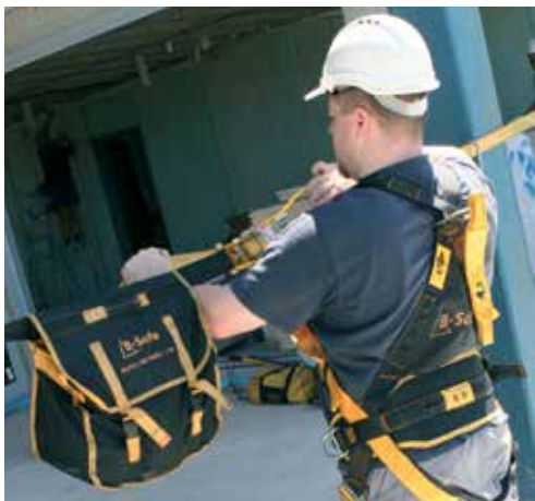
Web temporary life line, ratchet tensioning method.
